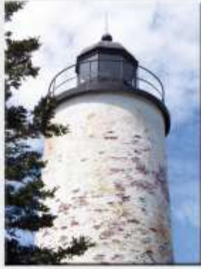
Baker Island Lighthouse
