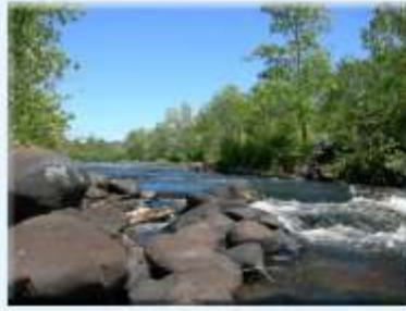
Copper Mine Dam
