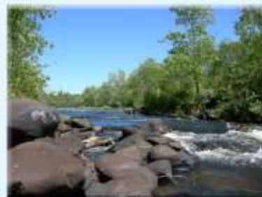
Copper Mine Dam
